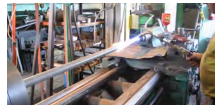
Spray & Fuse on Boiler Tubes
